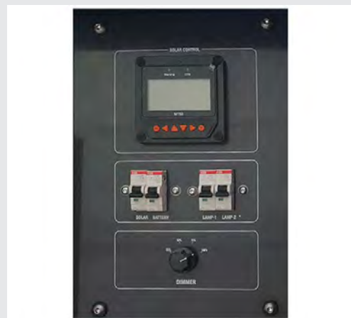
System Control Panel
